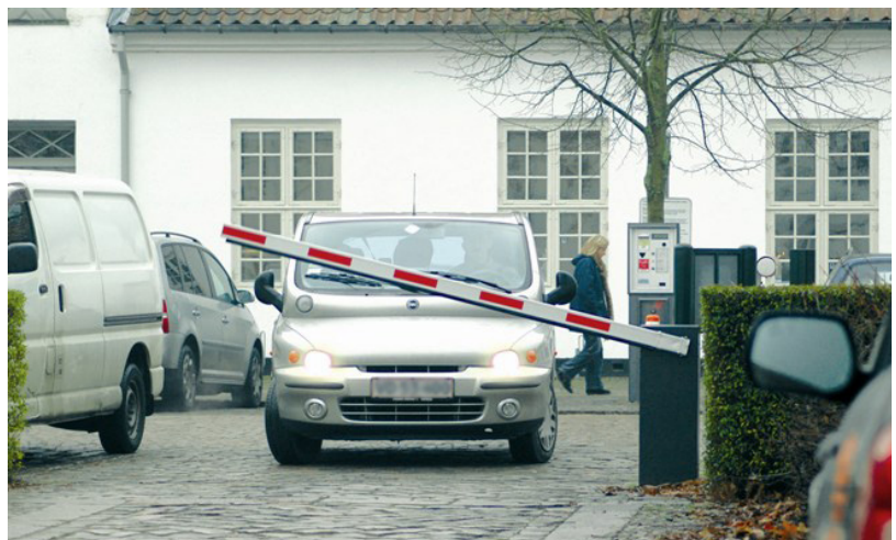
The parking bar opens when the predefined button is activated by touching the remote control reader.
